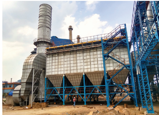
Reverse Pulse Jet Bag Filter with ID Fan and Blower specifically designed for the cement industry.
