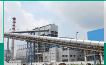
M/s. Bharathi Cement Corporation Ltd., Coal Handling System Tonnage: 3000 MT
