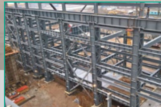
M/s. Nirma Ltd. TG Building Structures Tonnage: 4000 MT
