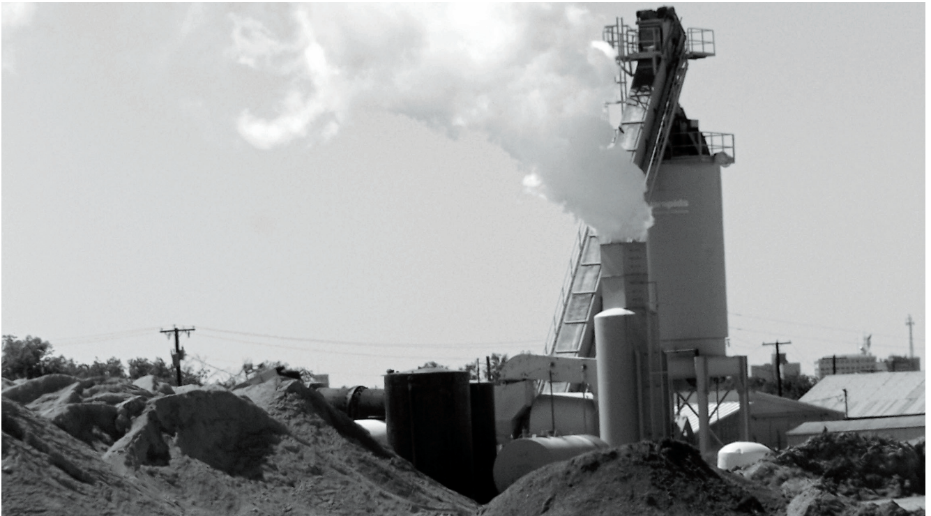
Exposure to cement dust may lead to health hazards for workers like respiratory issues, and skin and eye irritation.
